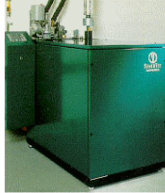
Reciprocating Cogeneration Engine Unit (SenerTec)
