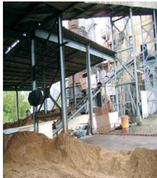
Picture After Modification
