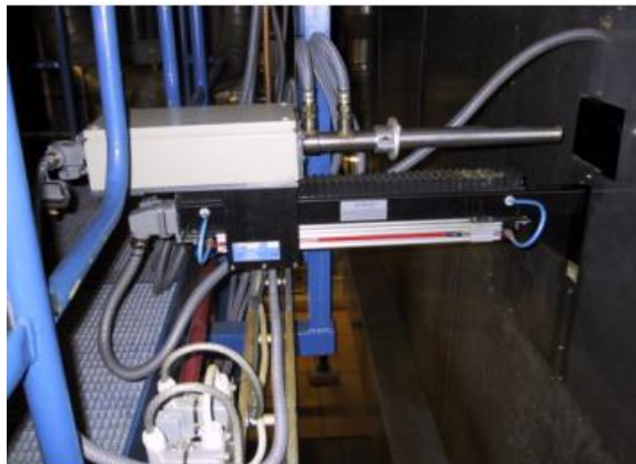
PiT Multisensor with pneumatic retraction system on a 220MW coal fired boiler
