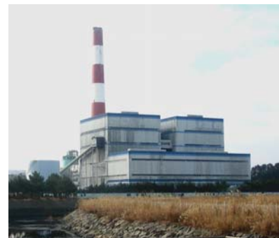
KEPCO, Power Plant Seocheon Seocheon, South Korea (2 Units) 220 MW
