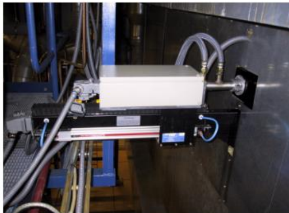
PiT Multisensor with pneumatic retraction system on a 220MW coal fired boiler
