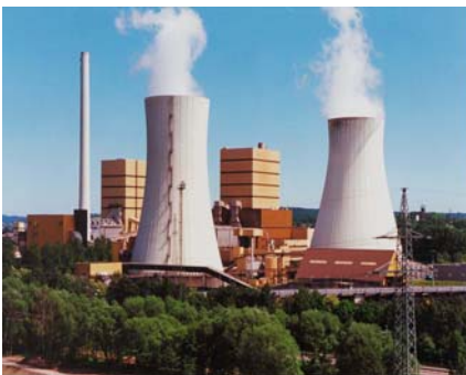
RAG Saarenergie, Power Plant Fenne Völklingen, Germany (1 Unit) 230 MW
