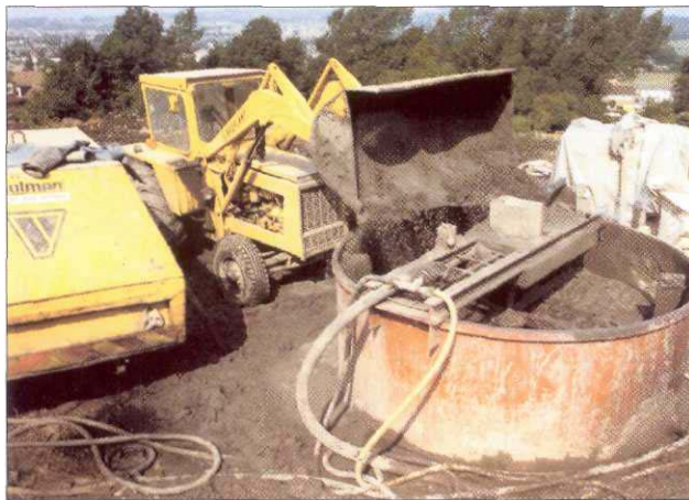
Figure PFA mixed into slurry form
