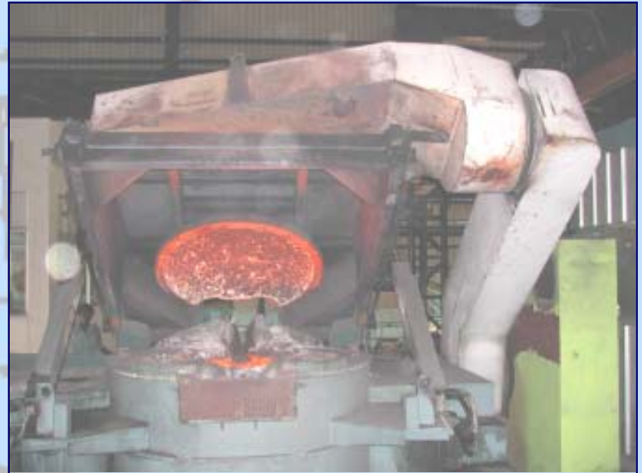
Furnace with closed capture hood
