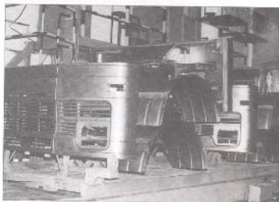
The skid that now accommodates 4 cowl instead of 2
