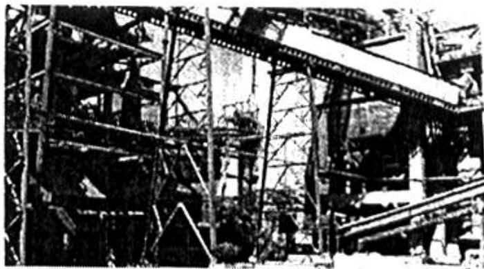
Fig : Transfer System of crushed clinker from CM-2 roller press to CM-1
